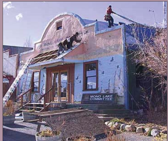
The new roof on the Mono Lake Committee headquarters.
