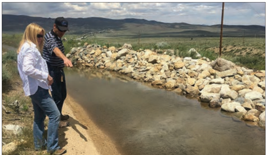
The Mill Creek return ditch is a critical piece of infrastructure used to return water back to Mill Creek after it passes through SCE’s hydropower plant.
