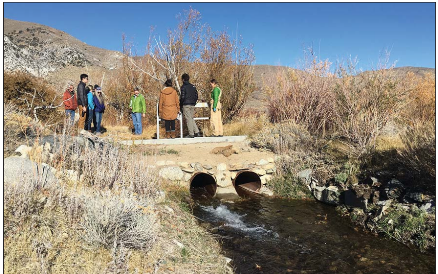
The Mill Creek return ditch carried flows of up to 16 cubic feet per second during a 61-day test last fall, returning water to the creek consistent with long-established water rights.
