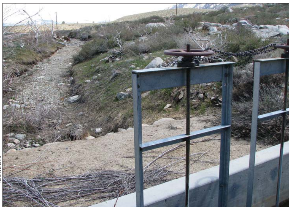
The hundred-year-old Mill Creek return ditch—soon to be a buried pipeline.
